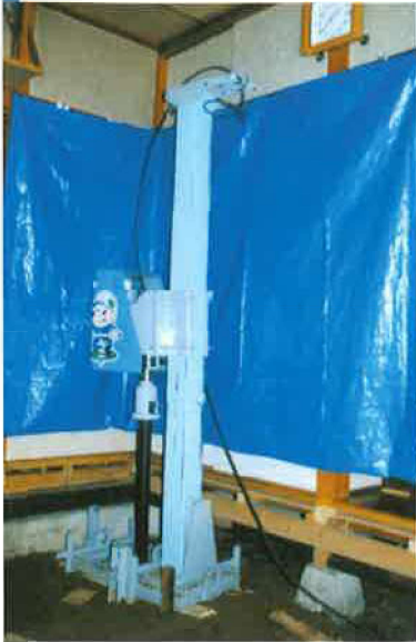
Subsidence reinforcement while residing in the building
