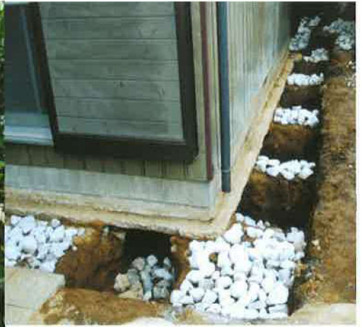
Reinforcement of the foundation after constructing with the Home pile carry
