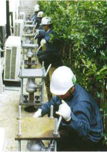
Jack-up for subsidence correction
